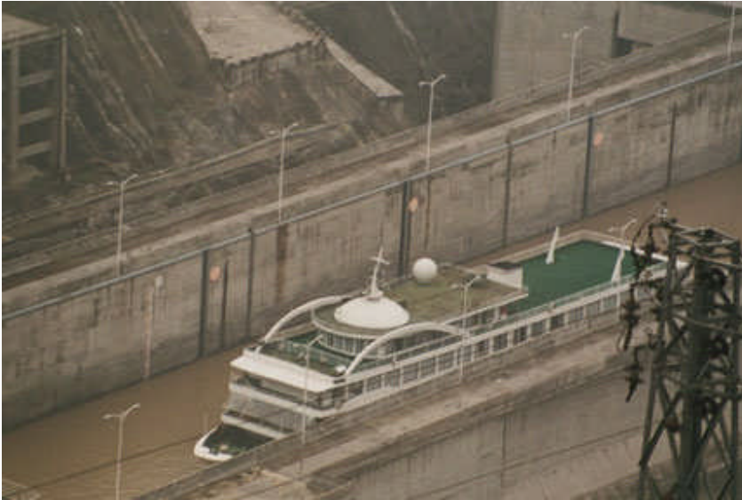
Tourist-toting riverboat in one of the Three Gorges Dam’s shiplocks. (Claire Walter photo)
